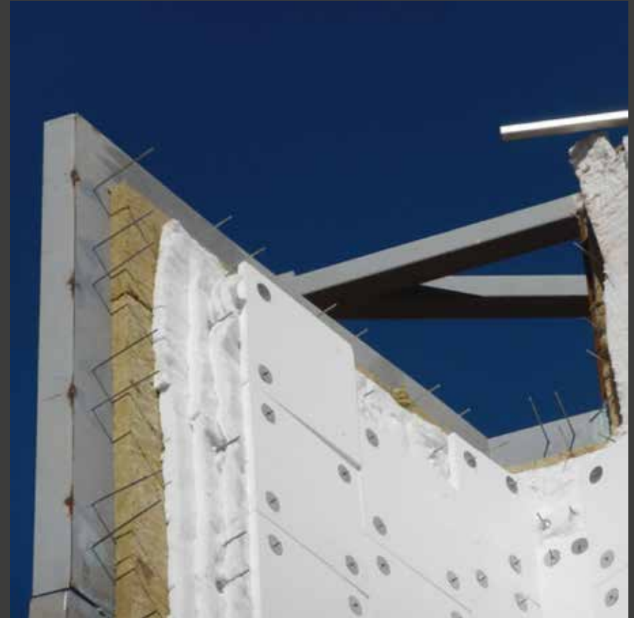
(Solar Power Plant - South Africa)
