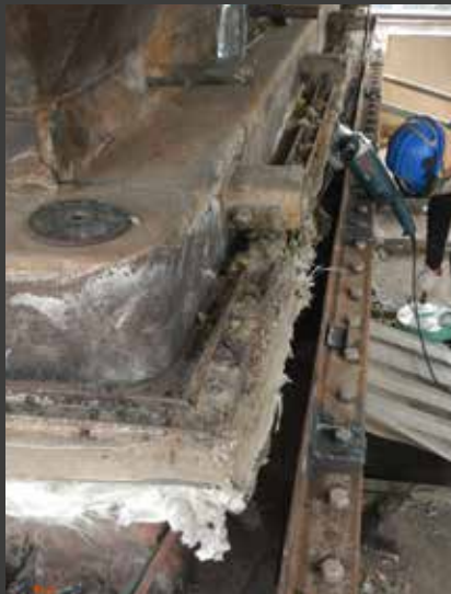
Removal of damaged existing one
