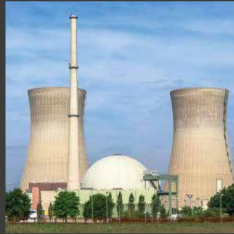
Nuclear Power Stations
