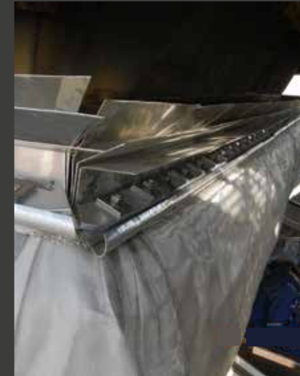
Erection of the new expansion joint
